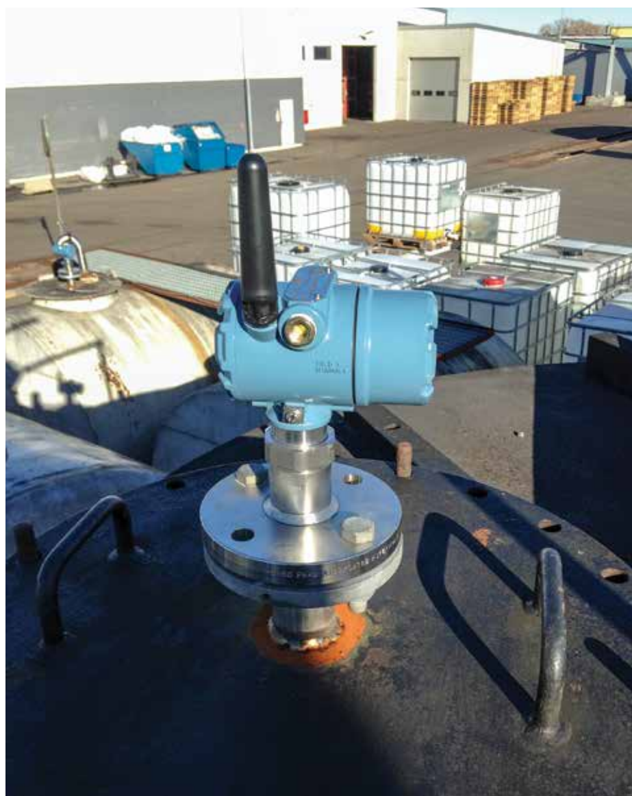
FIG. 2. A battery-powered WirelessHART instrument requires no signal or power wiring, and no wiring support infrastructure.
